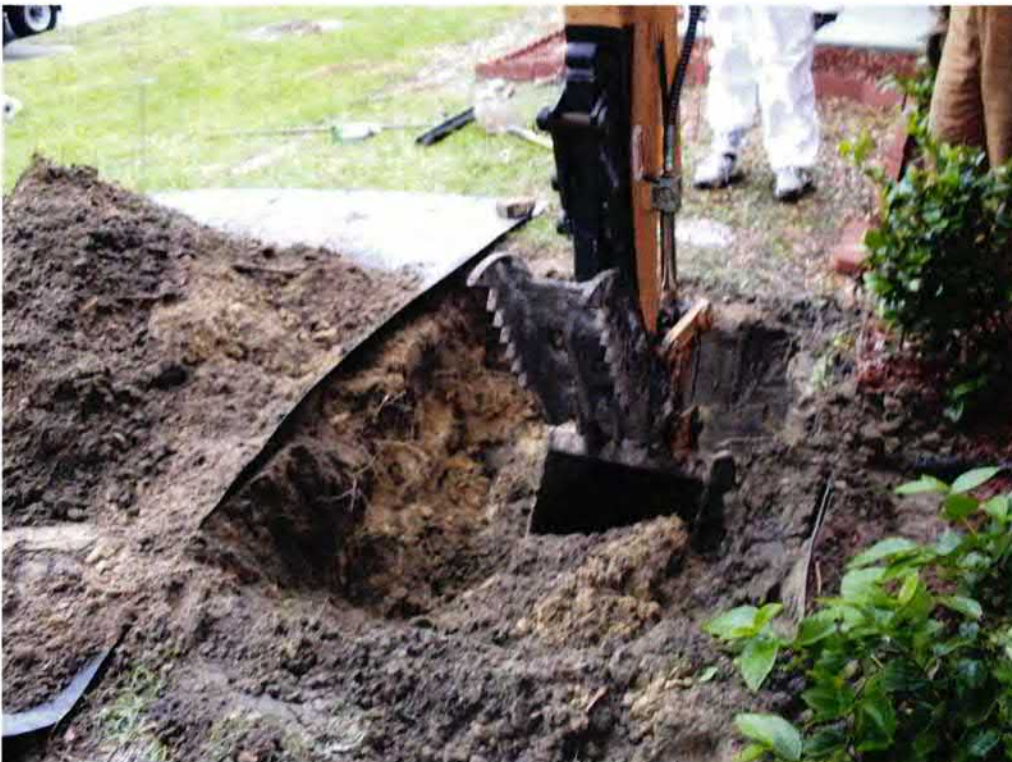
Picture 2: UST 572Dahlia excavation in progress.
